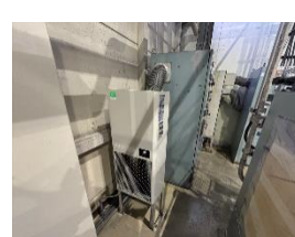
Replacing the panel cooler (after) Case 5 (CoorsTek Tokuyama)
